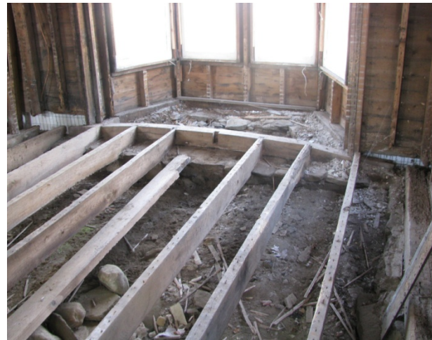
Crumpling field stone foundation
