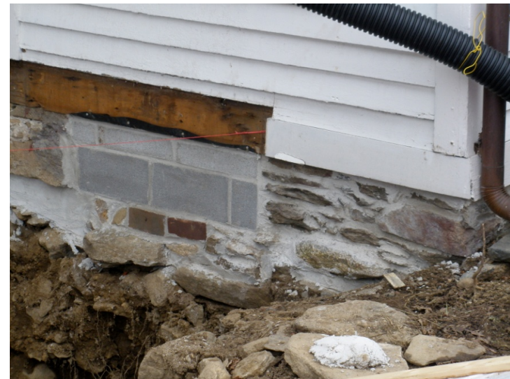
Deteriorated foundation being repaired
