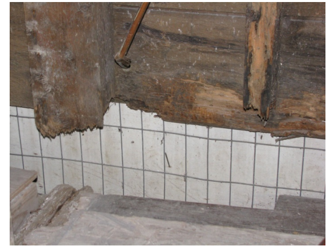
Rotted sill, damaged posts + beams
