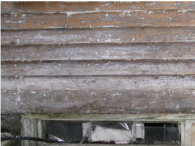
Damaged windows, rotted frames, worn chipped paint, damaged shutters
